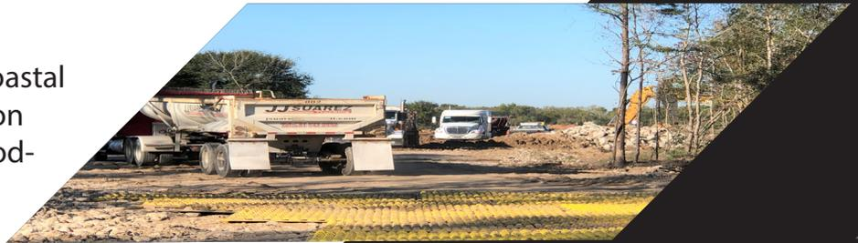
projects to explore techniques to control sediment and erosion on construction exits. The FODS construction entrance BMP was demonstrated to reduce street sweeping by 59% compared to traditional construction entrances. In addition, a reduction in required maintenance frequency allowed
