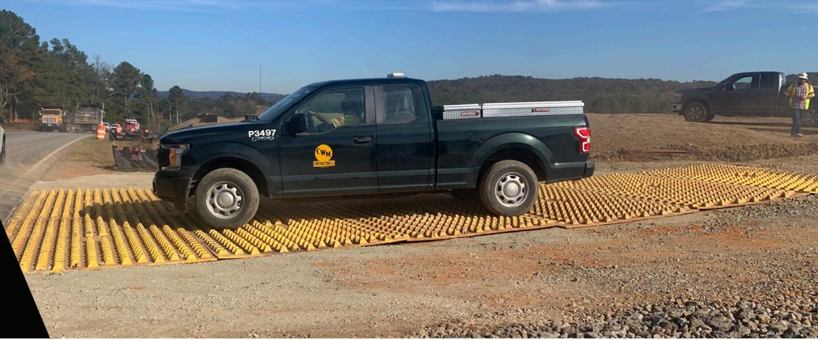
Linear highway projects often require tens or hundreds of entrances as contractors move through each phase of work. When choosing a construction entrance solution, contractors and engineers must explore solutions that minimize tracking, are cost effective over the full scope of the project, and minimize roadway hazards.
