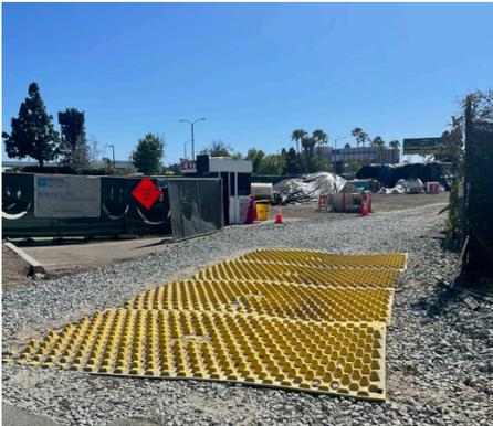
FODS Replacing Aggregate Exit
